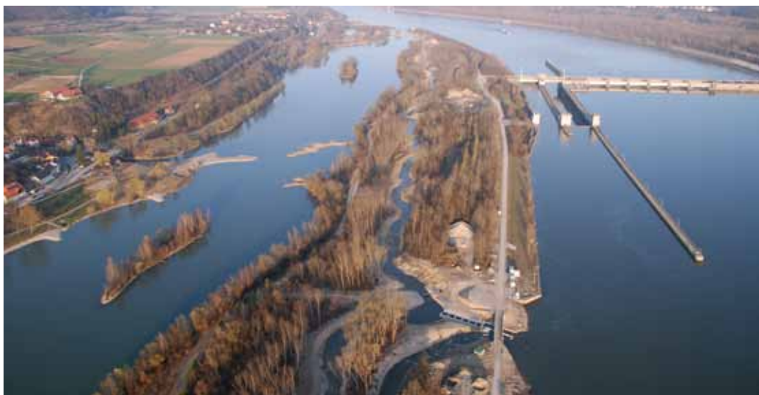
Aerial view of the 2 km-long fish pass constructed by the Donau-Ybbs project
