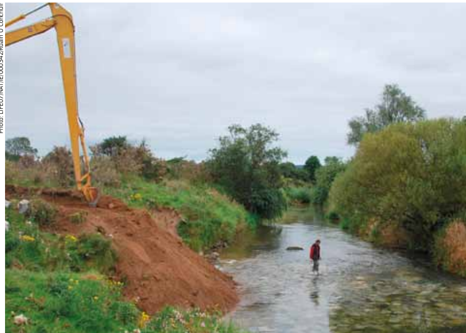
Inspecting a newly-constructed rubble mat (instream work) on the Mulkear River
