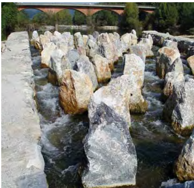
Fish pass near Sarzana railway bridge. The project found that sea lampreys prefer passes with boulders in a grid pattern
